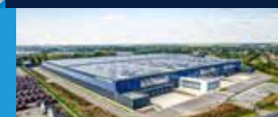
Panattoni Park Paris North 📍 Beauvais 45 000 m 2
