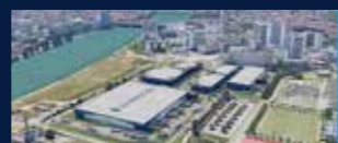
Panattoni City Dock Triborder 📍 Basel 43 000 m 2
